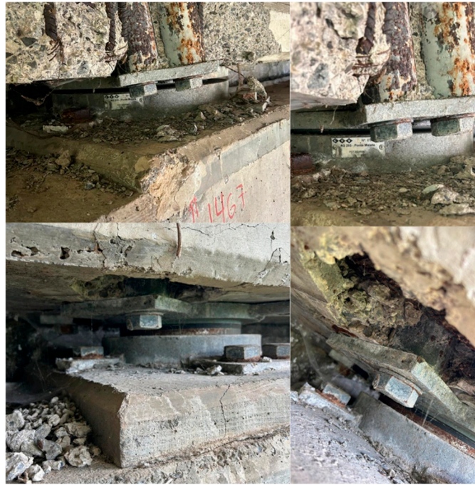
Figure 12. Close-up view of the two bearing elements on the northern pier.
