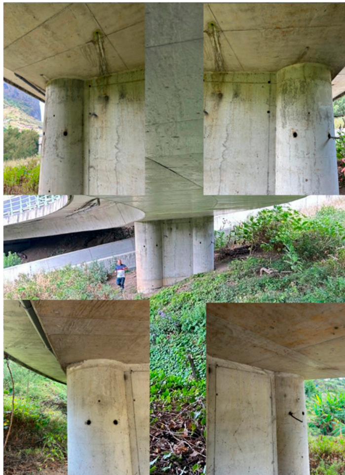
Figure 13. View of the bridge's central pier, in excellent condition.
