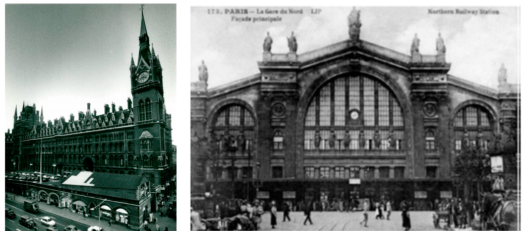
Figure 1. The façade of St. Pancras station (left), with the hotel building covering the central nave, and the façade of the Gare du Nord (right), with the geometry of the inner nave facing the outside. Source: Aróstegui.
