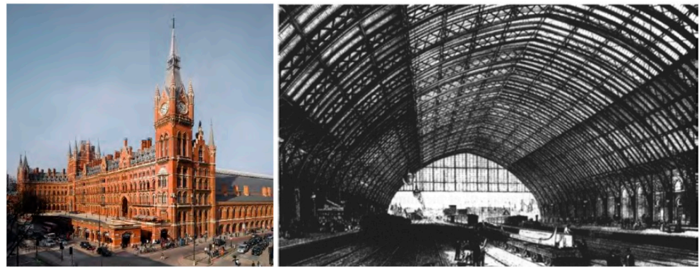
Figure 7. St. Pancras Station. Photograph of the exterior of the Midland Grand Hotel (left) and photograph of the interior of the station in 1870 (right). Source: Aróstegui.
