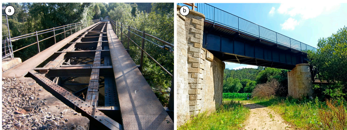
Figure 3. Views of the bridge: (a) during rehabilitation works and (b) after rehabilitation works.
