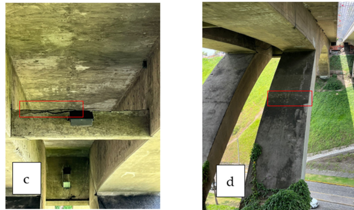
Figure 2. Structural cracks and fissures detected in a previous visual inspection. (a) Crack identified under bridge deck. (b) Crack identified under bridge deck. (c) Crack identified in cross-beam. (d) Crack identified in arch.
