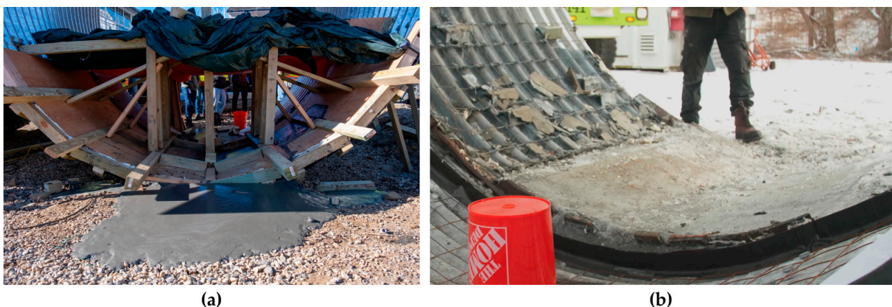
Figure 15. (a) UHPC spilling out of wood formwork; (b) final cast after demolding.
