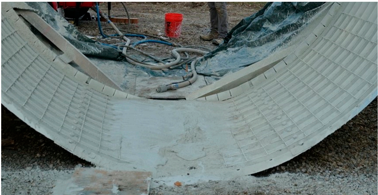
Figure 18. Final shotcrete UHPC cast showing pooling at the bottom and minimal build-up on the culvert walls.
