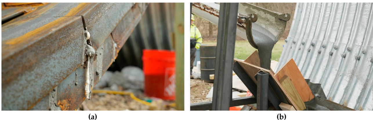
Figure 11. (a) Steel angle bulkhead showing minimal UHPC leakage; (b) ready-mix truck dispensing UHPC directly into bird's mouth funnel.
