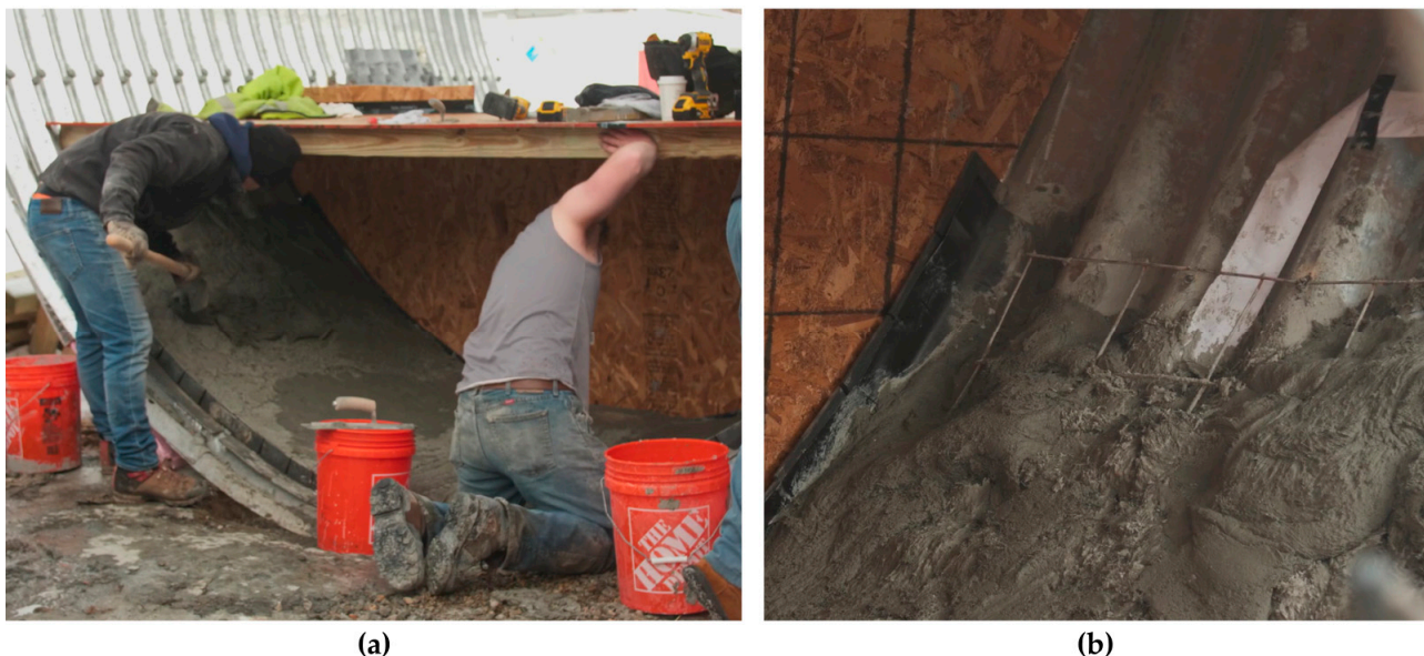
Figure 12. (a) Hand troweling thixotropic UHPC into culvert; (b) UHPC build up and surface over wire mesh.
