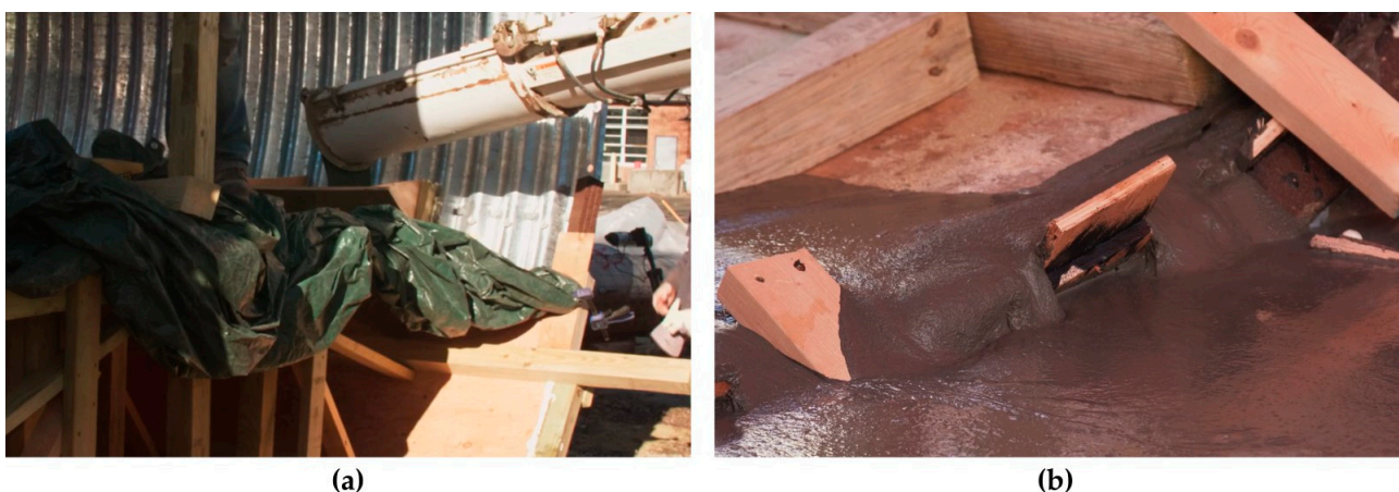
Figure 8. (a) UHPC cast directly from ready-mix truck into bird's mouth on one side of the formwork; (b) UHPC spilling out of the formwork through split bulkhead seal.
