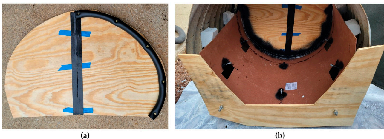
Figure 4. (a) Keyed formwork with hinge in the middle; (b) completed formwork.
