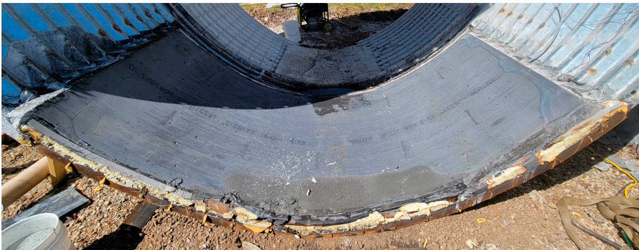
Figure 16. Final steel formed UHPC cast showing consistent thickness and surface.
