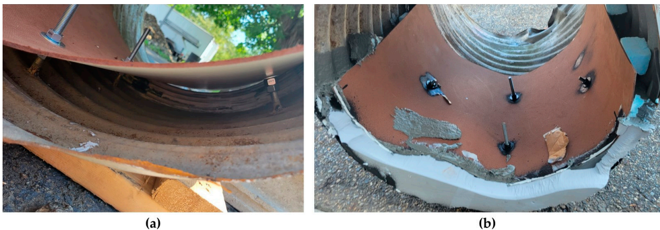
Figure 3. (a) MDF board with standoffs and 2-inch gap; (b) completed, sealed formwork showing standoffs and bulkhead.
