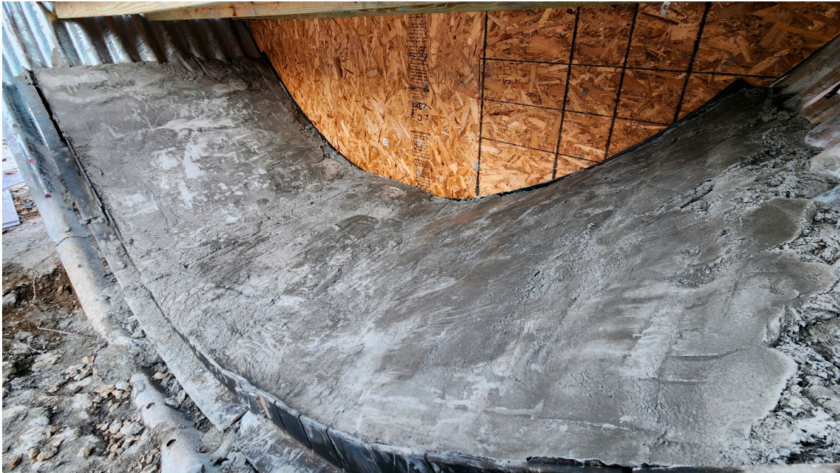
Figure 17. Final thixotropic UHPC cast showing consistent thickness and rough surface.
