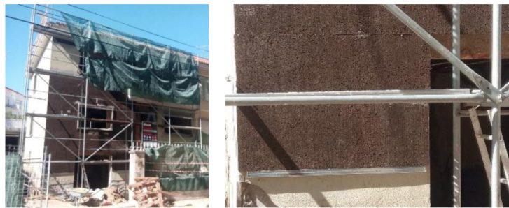
Figure 4. ETICS with ICB (insulation cork board) application (case D).
