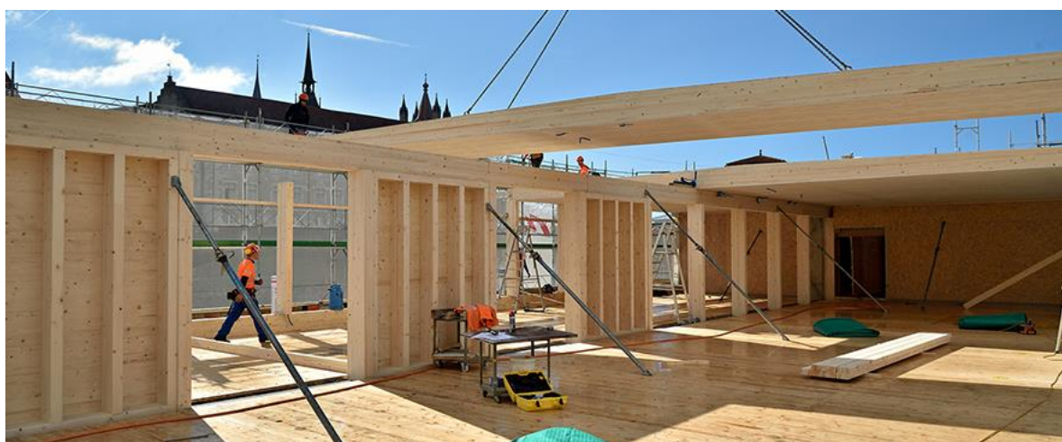
Figure 8. On-site assembly of the prefabricated wooden elements.
