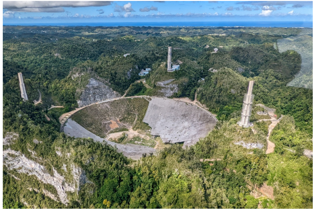
Figure 4. Aerial image of the Arecibo telescope during demolition, following its collapse. The instrument platform was suspended by a system of cables (see Figure 2) and fell into the dish, causing significant damage to the structure. Photograph by Tedder, distributed under a CC-BY 4.0 license.
