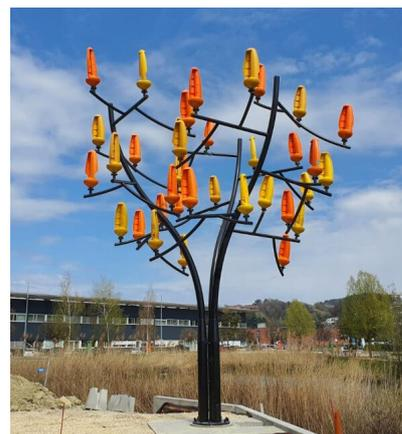
**Figure 2.** Technical specifications of the Windtree and WindTree is a steel structure (trunk and branches) on which 36 Aeroleaf<sup>®</sup> were installed. Reprinted with permission from [57], Copyright© 2024, New World Wind.
