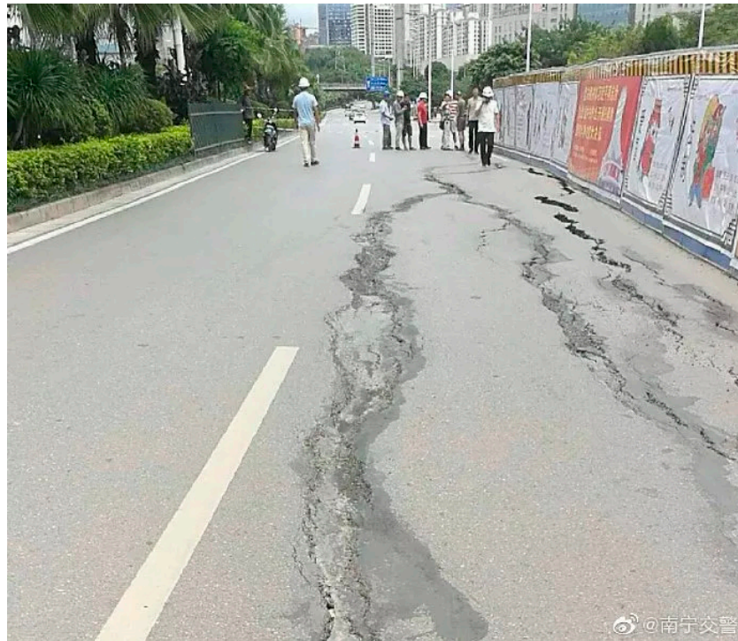
Figure 2. Cracks on the surface of Dongge Road prior to the incident (source: https://mp.weixin.qq.com/s/nMGCnVwHjIqVq_np9ITXwg ).
