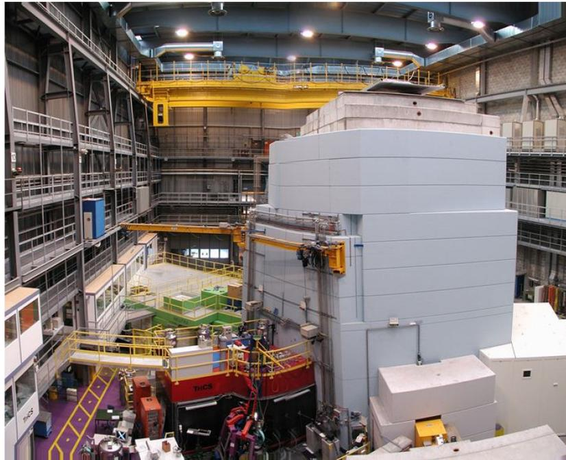
**Figure 8.** Overview of the SINQ installation; the green area on the left side is the NEUTRA imaging facility, where the NEURAP experiments have been performed, NEURAP is placed from the roof.
