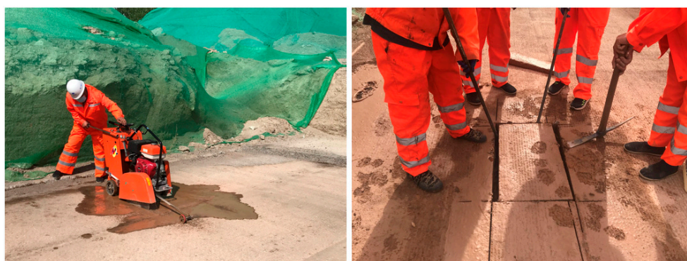
Figure 21. Schematic of the cutting and sampling process.
