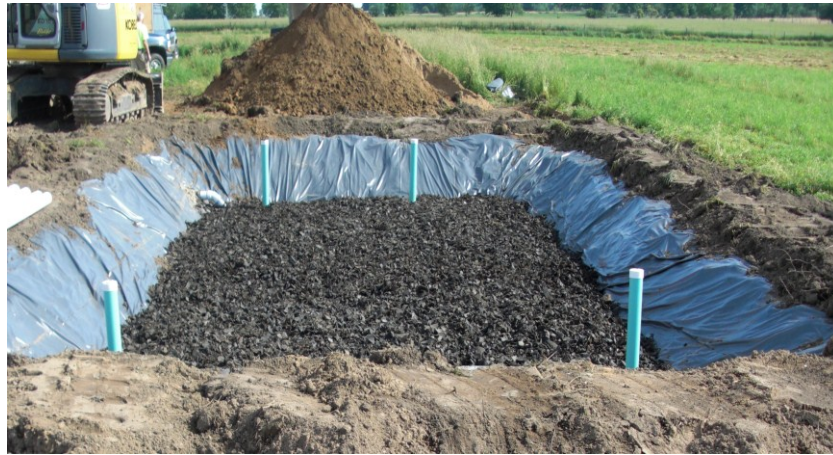
Figure 3. Front view of the constructed wetland cell showing the shredded-tire chips.
