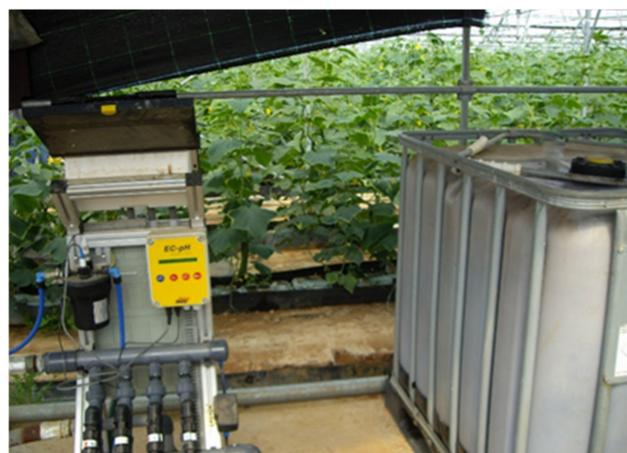
**Figure 3.** Groundwater supply pump (a) and an irrigation control head unit (left-hand side; b to d) consisted of a water meter (b); a filter (c); a fertiliser injector unit (d); electric valves (e), and a fertigation head used for soilless cucumber production in Mediterranean greenhouses (right-hand side).
