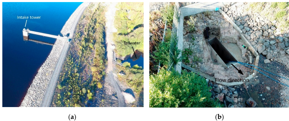
Figure 1. Bottom outlet in question: (a) intake tower in front of the embankment dam and conduit exit in the tailwater; (b) the exposed conduit exit during planned maintenance when the tailwater is drained (photos by HydroTerra).
