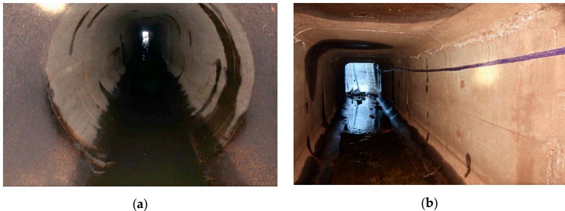
Figure 4. Horizontal conduit when emptied of water during an inspection: (a) a short section of a circular conduit (diameter 2.55 m), looking upstream towards the bend; (b) a major rectangular conduit with four rounded corners (2.55 m in width, 2.55 m in height), looking downstream towards the exit.
