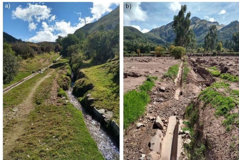
Figure 6. (a) A modern concrete canal with control gates adjacent to an earthen canal. (b) Destruction to concrete canal following March 2019 debris flow.
