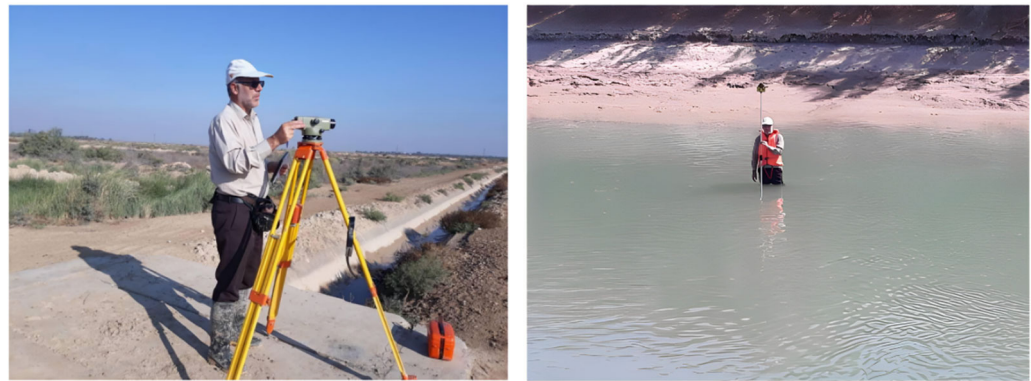
Figure 2. Examples of field surveying activities illustrate topographic mapping and spatial data collection along the river and traditional channels.
