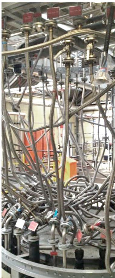
**Figure 2.** Flexible hoses as interconnections between fixed equipment piping in a multi-purpose-plant coupling station of Lonza AG.
