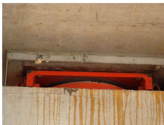
**Figure 9.** A lead rubber bearing on Yingzhou Bridge.
