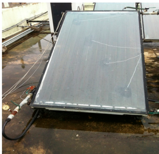
Figure 8. Photograph of thermosyphon solar FPC.
