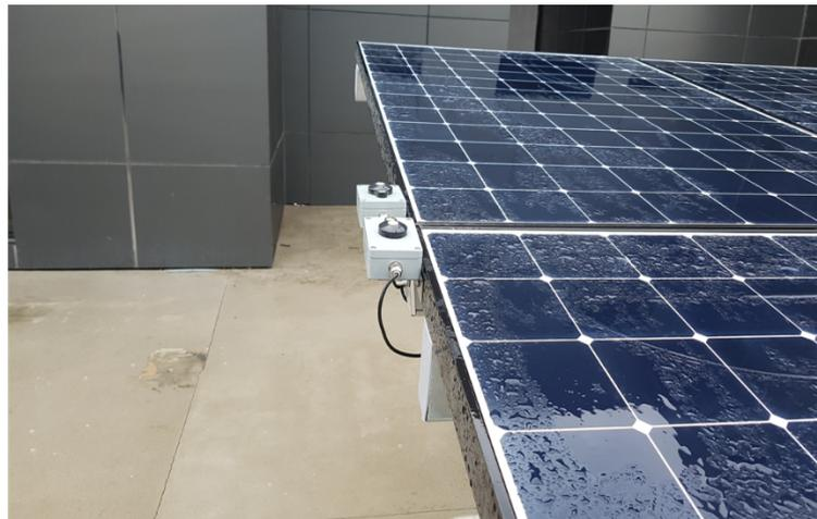
(a) Environment sensor and PV panel.
