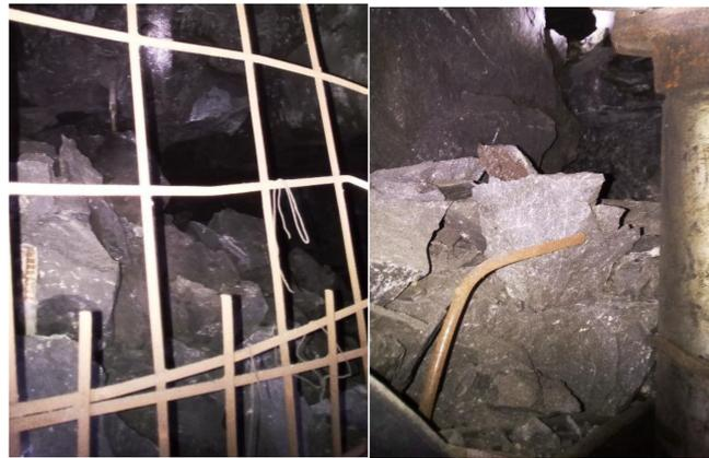
Figure 1. Fractured porous rock mass.
