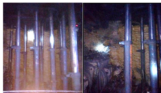
Figure 3. Construction of gangue bag separation wall.
