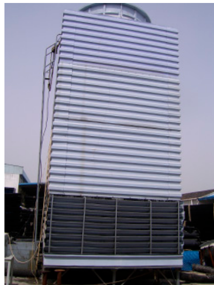
Figure 5. Pictorial diagram of the test shower cooling tower.
