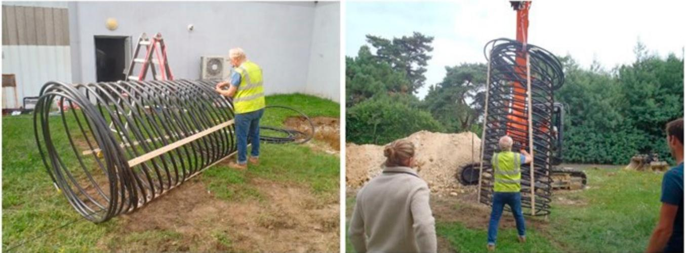
**Figure 1.** Installation of a spiral (earth basket) ground heat exchanger with a fibre-optic distributed temperature sensing system at the IUT Civil Engineering Student Laboratory (Bordeaux, France) pilot site (picture: Groenholland Geo Energy systems).
