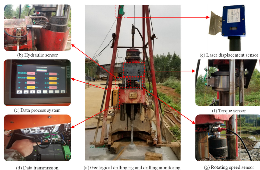
Figure 1. Digital drilling system and in situ testing.
