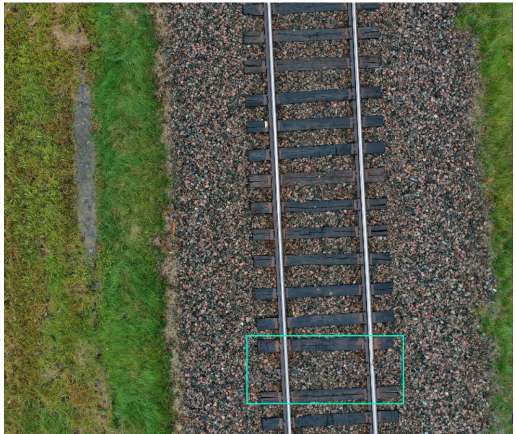
Figure 7. Example of a missing tie.
