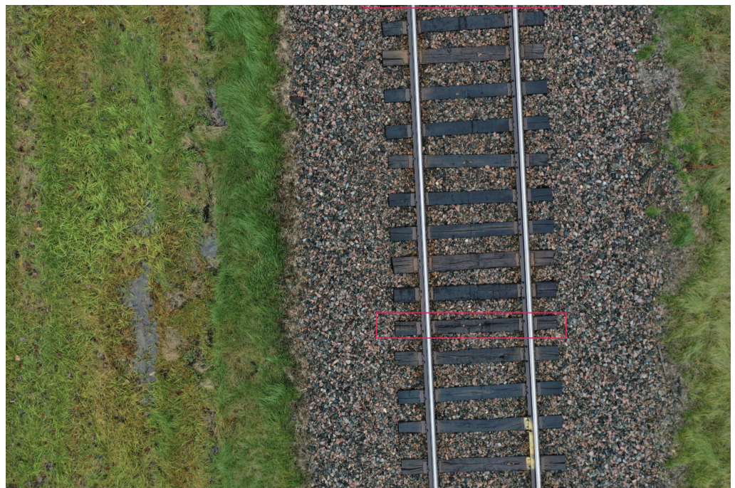
Figure 8. Example of a broken tie.
