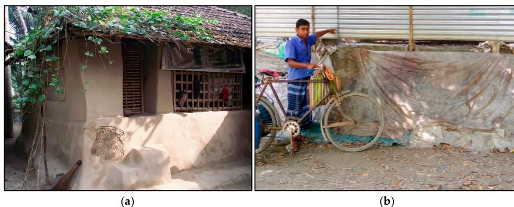
**Figure 4.** (a) Mud house with elevated plinth; (b) person denoting the flood water height in 2017 in Type 2 settlement (Image source: Authors).
