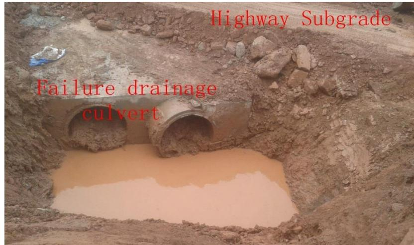
Figure 10. Drainage culvert failure at foot of slope.
