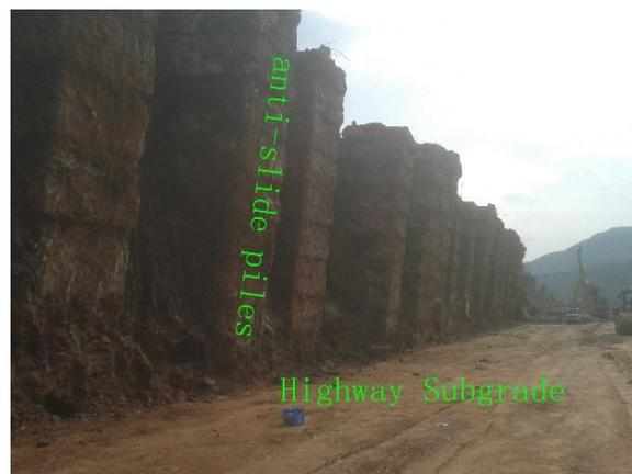
Figure 8. Anti-slide pile.
