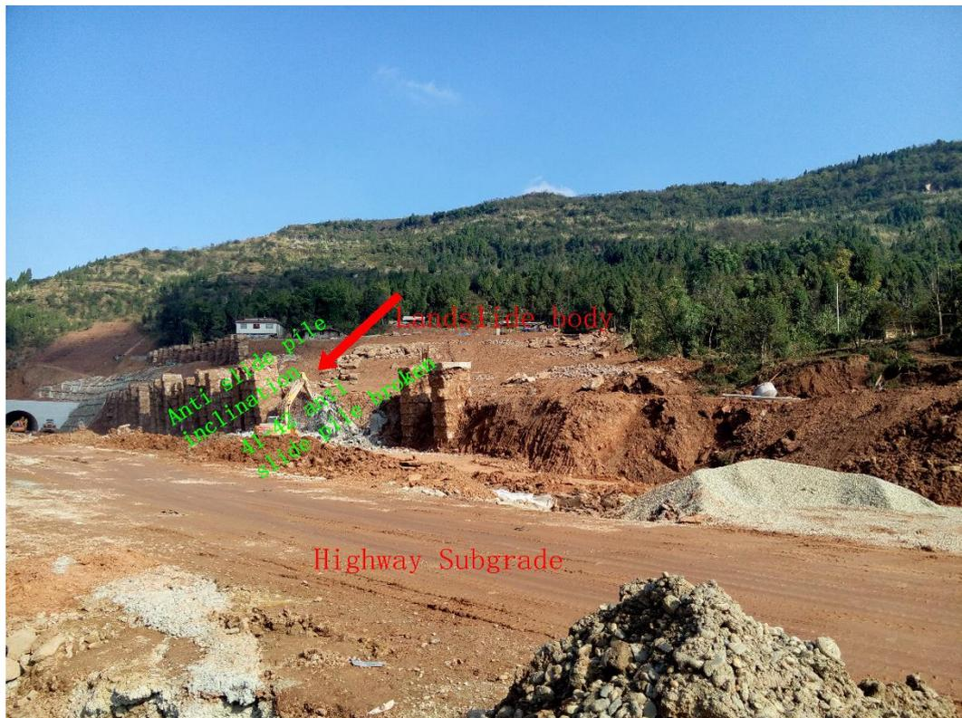
Figure 3. Fracture and inclination of the anti-slide pile.
