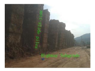
Figure 8. Anti-slide pile.
