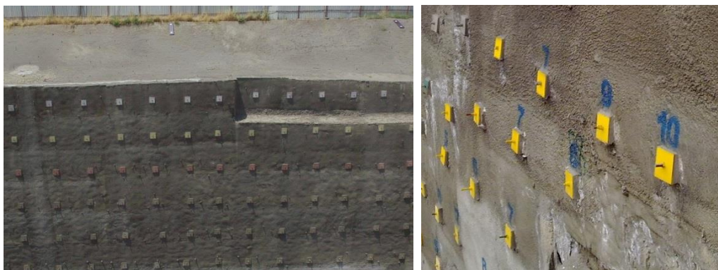
Figure 4. An example of wall nailing and the metal plate attached to the nails.
