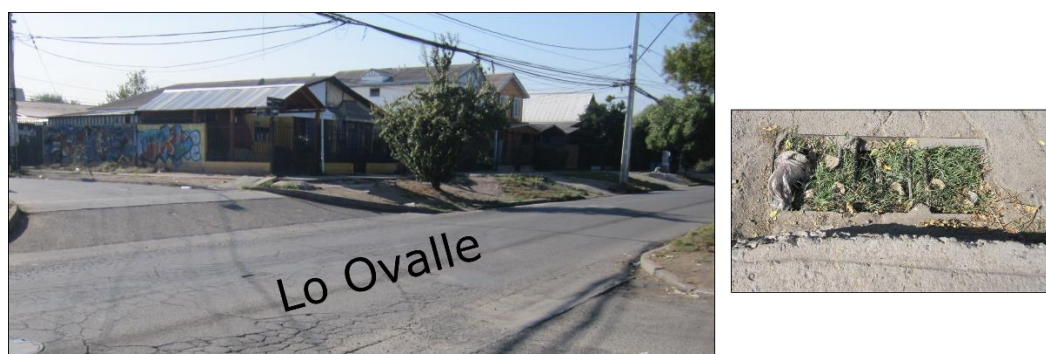
Figure 4. Quilicura: The street “Lo Ovalle” turns into a riverbed during rainfalls due to its lower level compared to the side streets. Blocked gullies increase the runoff (photos taken by author, Quilicura, 6 May 2015).
