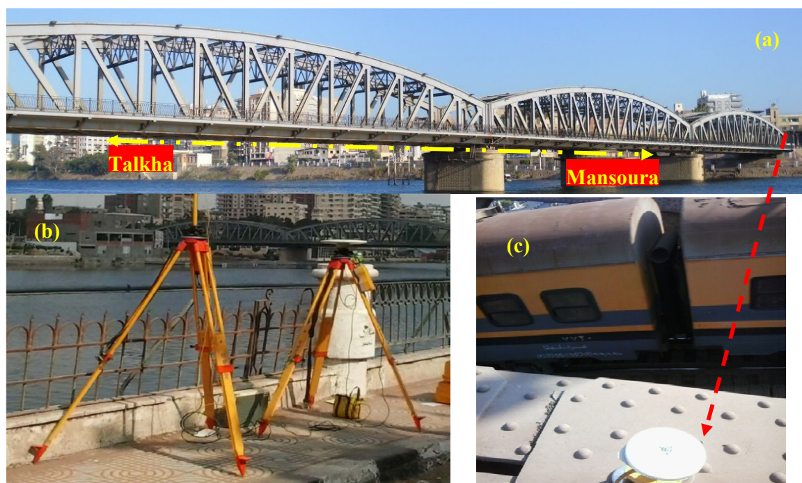
Figure 4. Mansoura Bridge and monitoring system: (a) bridge view; (b) base station GPS; (c) rover GPS.
