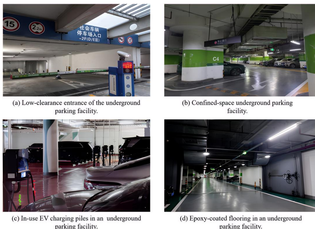
Figure 2. Fire incidents in underground parking garages. (the Chinese label “社会车辆停车场入口-2F(D/E区)” in (a) indicates the entrance to the public parking garage on Level 2F, (Zones D/E)).
