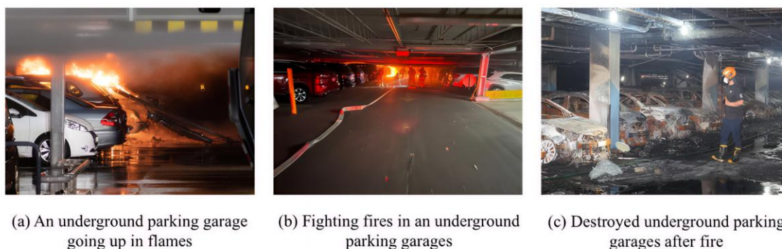
Figure 1. Fire incidents in underground parking garages.
