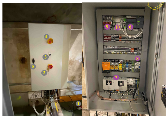
Figure 4. (Left): The control box of the new motion system for the FPSD detector. (Right): Inside of the control box with two inverters visible at the bottom and a Siemens PLC controller in the top right. Numbers in the figure explained in the text.
