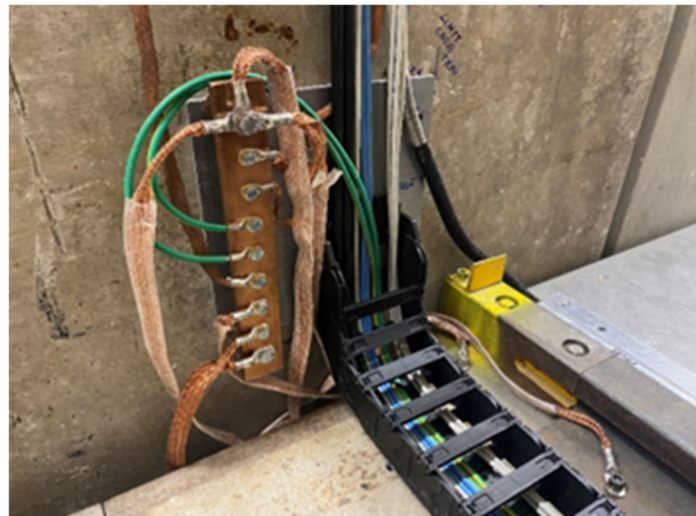
Figure 10. Central point of the grounding system.
