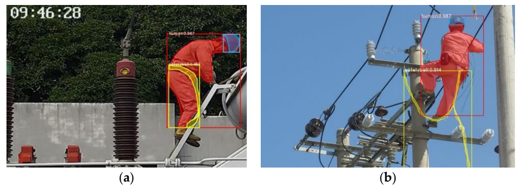
Figure 16. Detection for different working height (a) Construction on top of the main transformer (3 m high); (b) Construction on top of the telegraph pole (8 m high).
