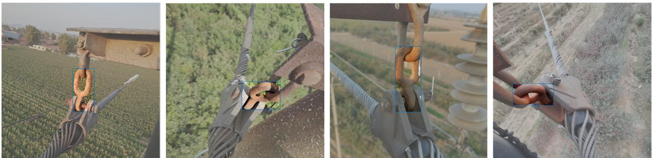
**Figure 14.** Visual results of detection of rusted fittings with UD-Net.
