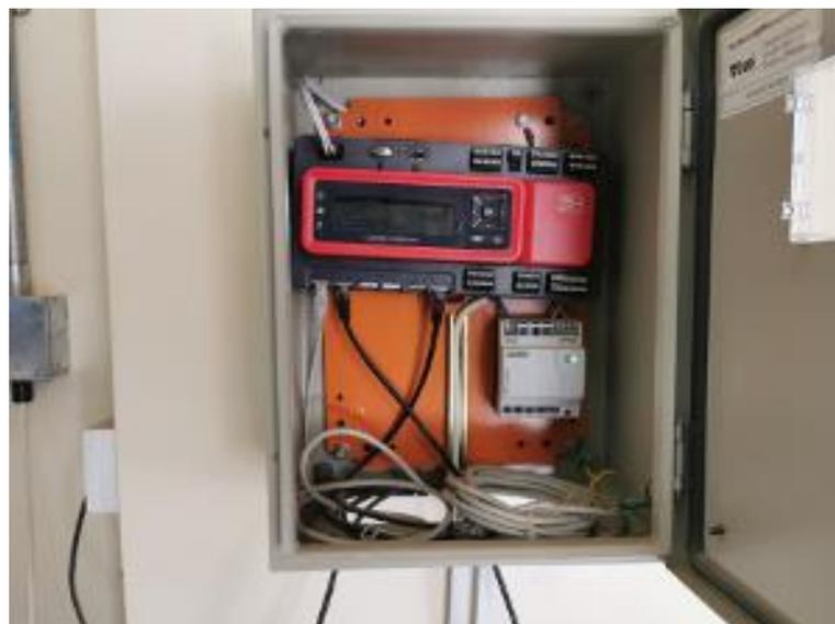
**Figure 10.** SMA cluster controller at the Solar Car Parking Station.
