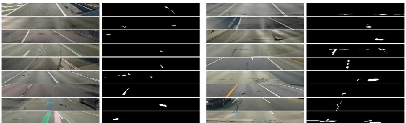
**Figure 4.** Examples of original and labeled images with road-surface cracks.
