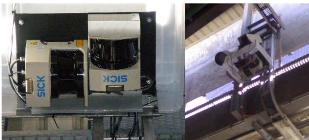
Figure 2. Overhead laser scanners mounted at a coal terminal dump station.
