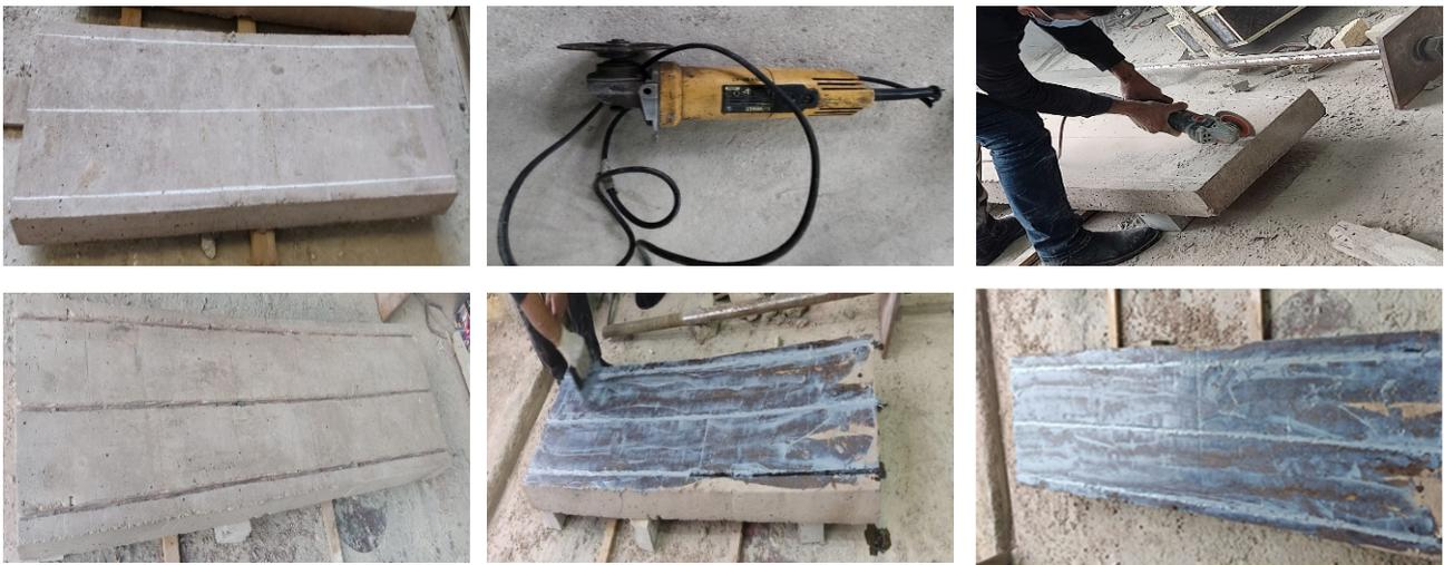
Figure 10. CFRP ropes installation.
