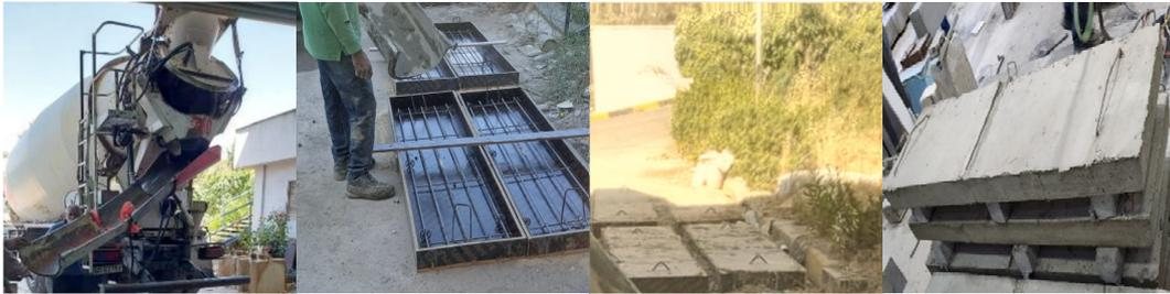
Figure 2. Slabs fabricated.
