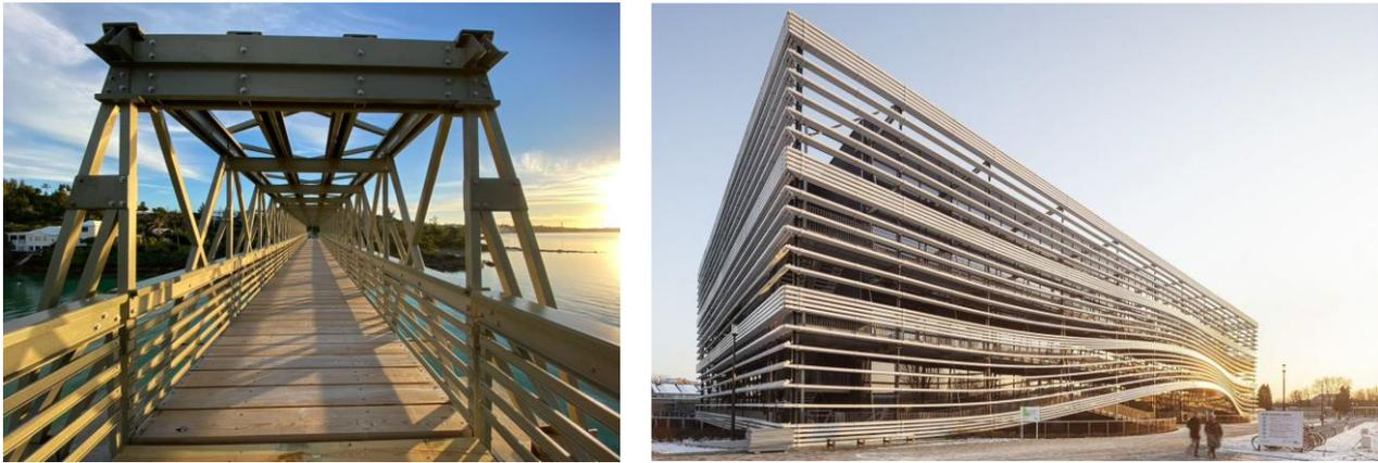
**Figure 2.** Composite pedestrian bridge in Bermuda (**left**) (Image courtesy of Creative Composites Group) and FRP profiles at the façade of a building on the University College Ghent's Schoonmeersen Campus (**right**) (Source: Open Oproep 2013).
