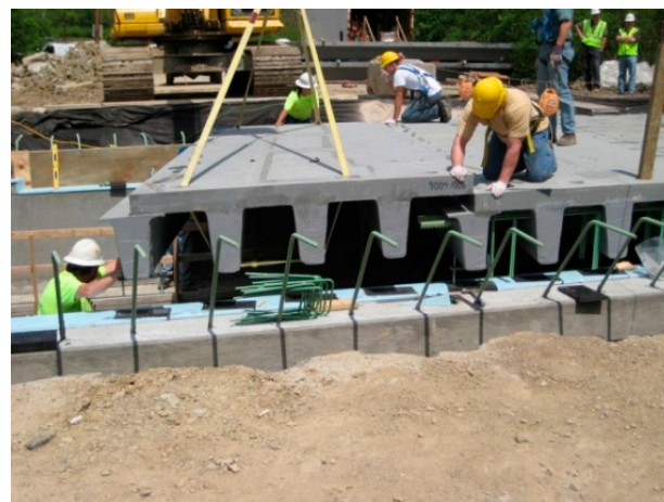
Figure 9. Installation of prefabricated elements of a SuperFiberSpan composite deck [52].
