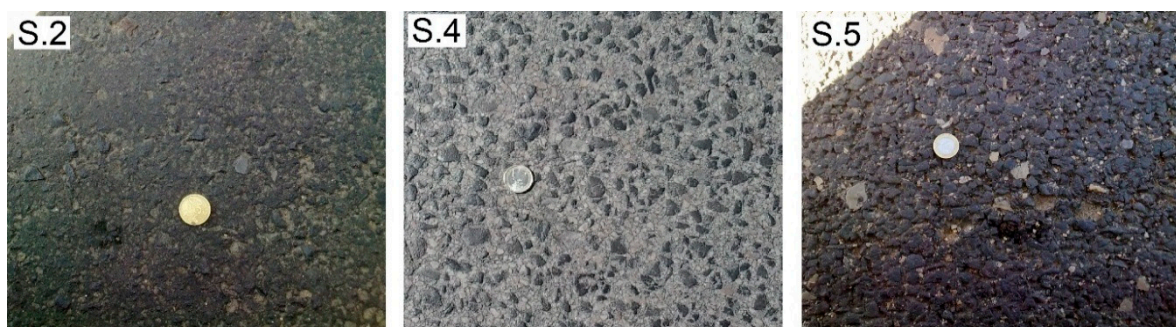
Figure 9. Comparison of some studied sections: S.2 (slurry seal), S.4 and S.5 (asphalt concrete)
