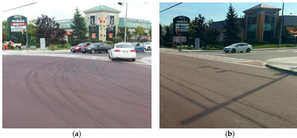
**Figure 7.** Tire marks at red asphalt sections paved by the Initial Red mixture: (a) newly paved section; (b) two-year-old section.
