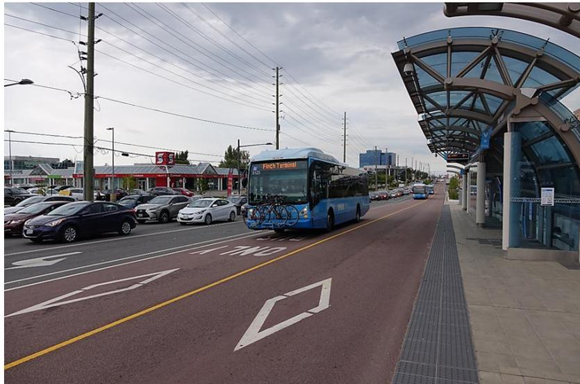
**Figure 1.** A section of coloured bus rapid transit (BRT) lane at York Region, ON, Canada.
