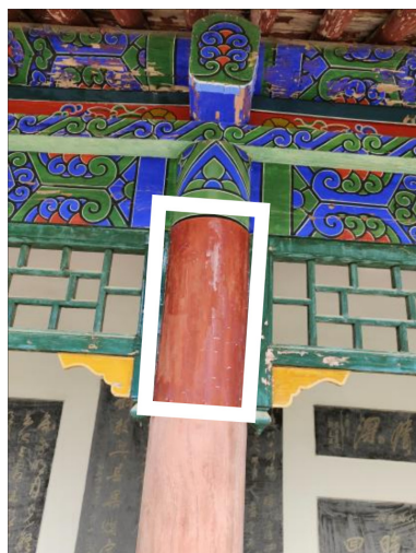
Apply protective coating (north side corridor of Zhaoren Temple)
