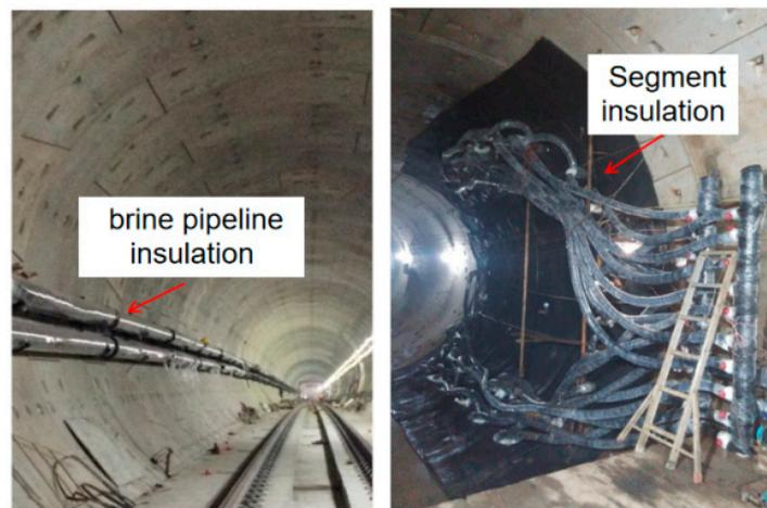
**Figure 9.** Heat insulation treatment of the brine pipeline and segment.
