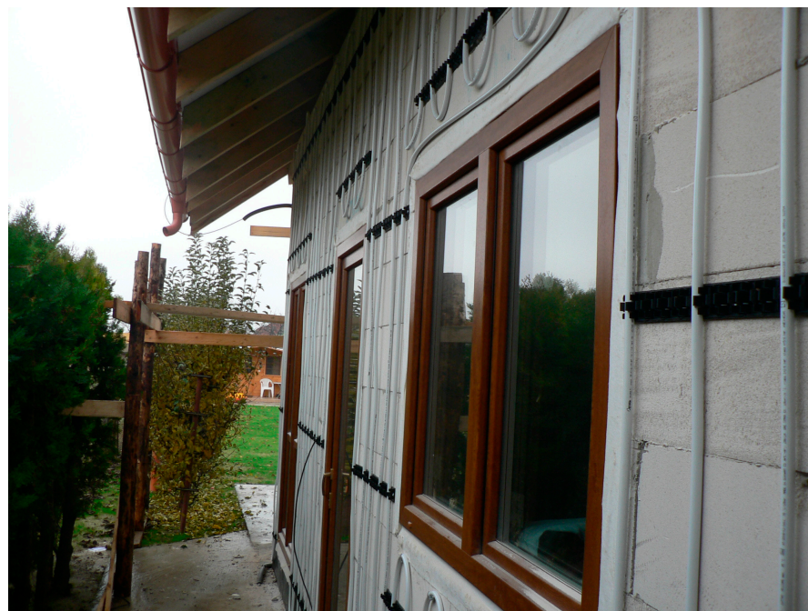
Figure 21. View of the ATP formed by a plastic pipe between aerated concrete masonry and polystyrene. (Photo archive: Kalús).
