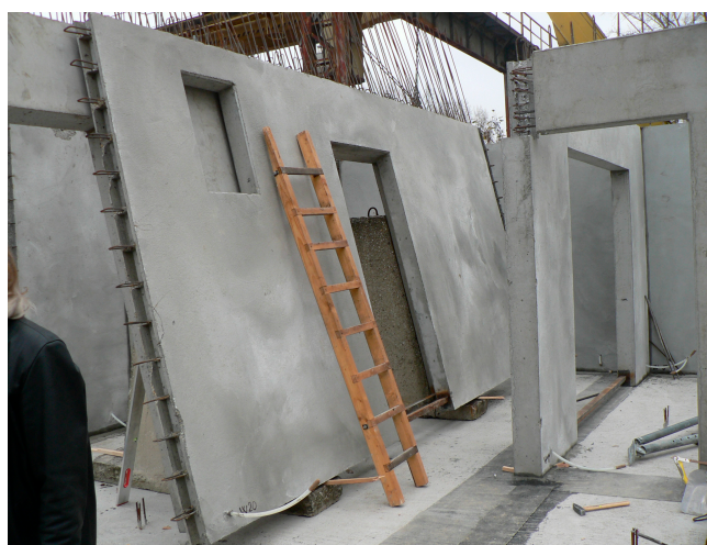
Figure 10. View of reinforced concrete panels with integrated ATP piping. (Photo archive: Kalús).
