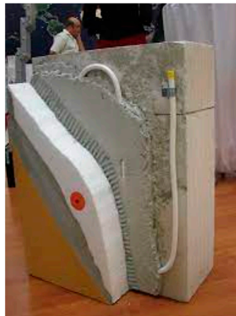
Figure 2. Application of TB on porous concrete block wall [5].
