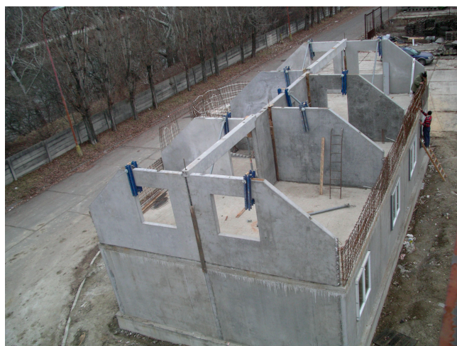
Figure 9. View of the assembly of the prototype prefabricated house IDA I. (Photo archive: Kalús).
