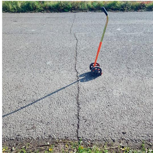
**Figure 14.** Recording road defects by visual inspection.
