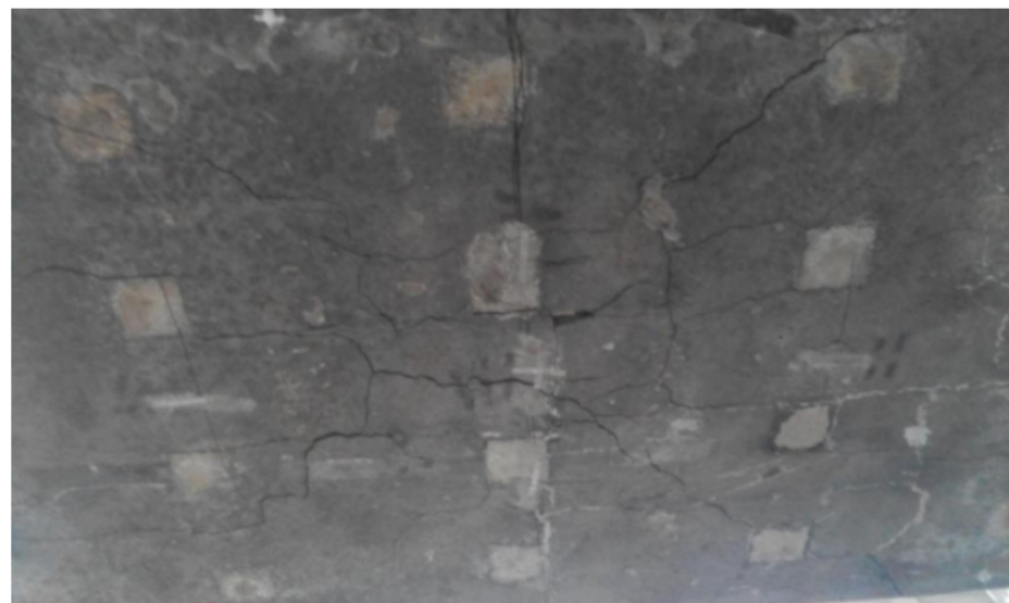
Figure 13. Failure of the precast bottom slab.
